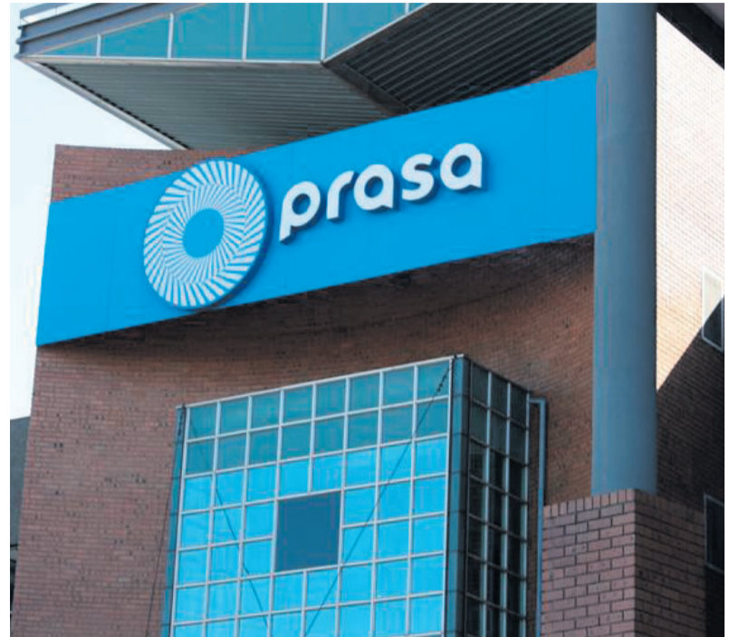
Security guards will protect Prasa infrastructure from vandalism and theft.
